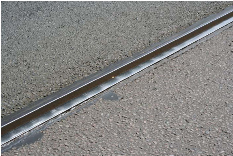
Fig 5. Example of a severe case of wave corrugations in the rail surface.
