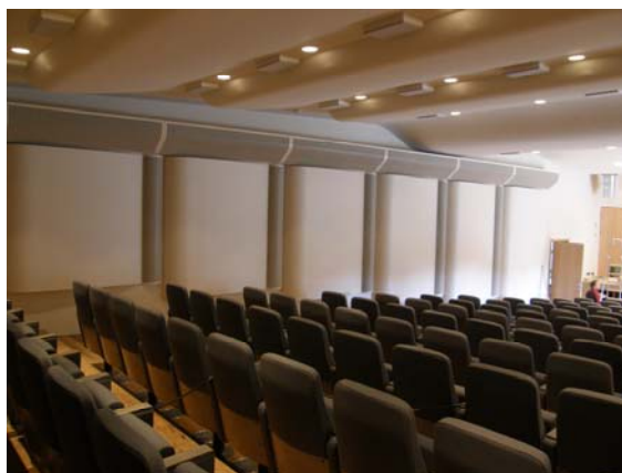
Figure 6: Seats in the hall, diffusers/reflectors on the walls with hidden loudspeakers- ceiling
